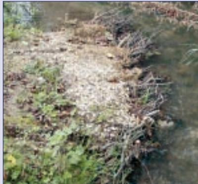
**Faggot Deflectors** were constructed from bundles of brushwood secured with timber pegs and wire and covered with locally excavated gravels.
