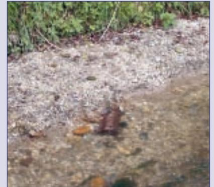
**Log Deflectors (Type 1)**, bedded on clay, secured with timber pegs and wire and back-filled with clay or gravel, were constructed from timber felled on site.
